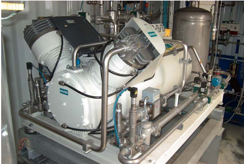
Oil-free two stage piston compressor VTOG 160/90 WM-W, water cooling, with gas tight magnetic coupling drive
