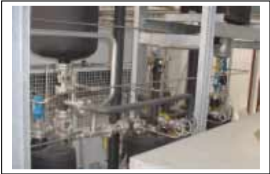
Gas reducer station and condensate collector
