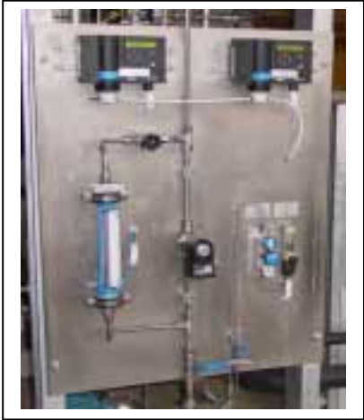
Gas reducer station and condensate collector
